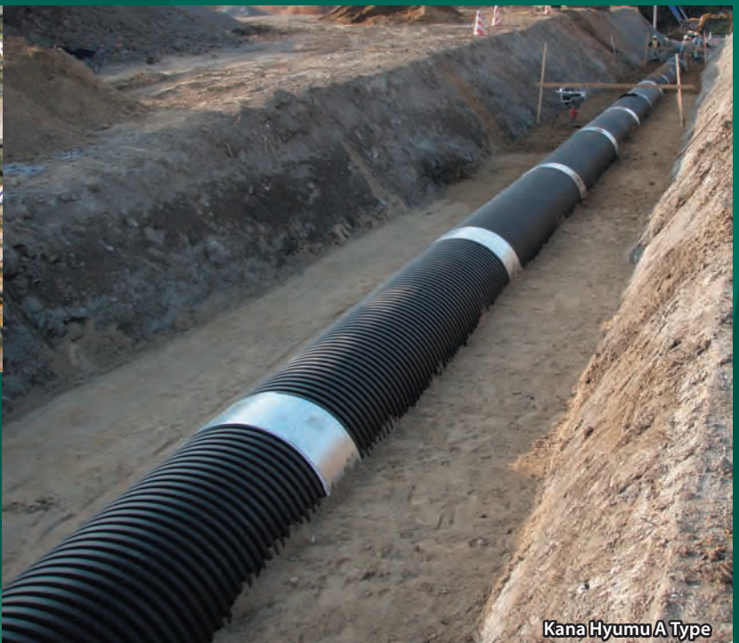
Kana Hyumu A Type With one-touch earthquake-resistance joint
