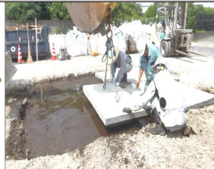
Place Kanacrete slabs on the ground
