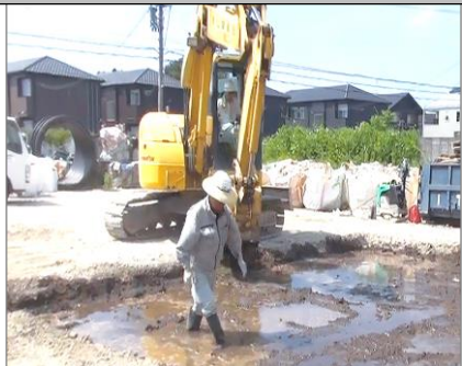
Preparatory work (Check the ground condition, etc.)
